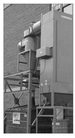
The cyclone separator is the most efficient dust collector for cost. These cyclones are equipped with top mount motors and fans, which pull contaminated air into the cyclone through the lower side opening. The centrifugal effect of the cyclone, created by rapid rotation of the high velocity air stream, forcibly precipitates dust out of the bottom and into a container, which fits the application. Clean air is released through the upper side opening.
